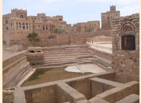
Picture (8.1): Typical traditional rainwater harvesting cistern from roofs
