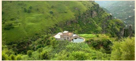
Picture (8.8) Traditional rainwater harvesting cistern at a house in the mountainous area in Yemen
