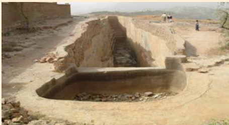
Picture (1.6) Rainwater harvesting Aljerroof
