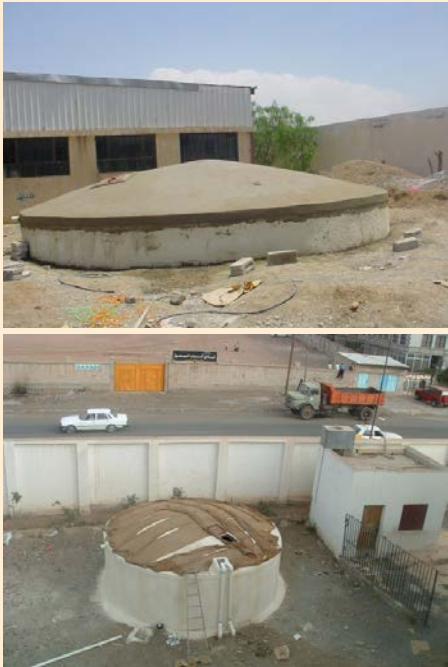
Photo (2) Two Ferro-cement tanks at two schools in Sana'a (Giz, 2007)
