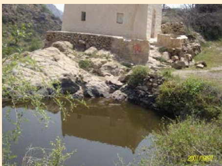
Photo (1) Rainwater harvesting from Mosque roof (traditional)
