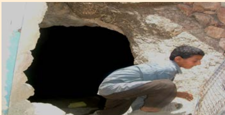
Picture (1.7) Kahf for underground rainwater harvesting
