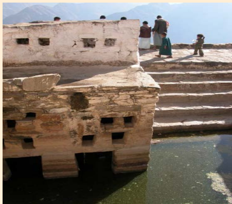
Picture (8.5a) Roof rainwater harvesting from a Mosque in Hajjah, Yemen ([19]
