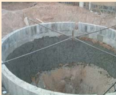
Picture (1.11a) Ferro-cement tank at a girls' school in Sana'a (during construction) (SFD)
