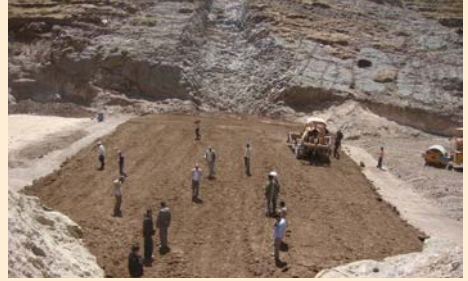
Picture (1.3) Natural foundation for Karef water harvesting
