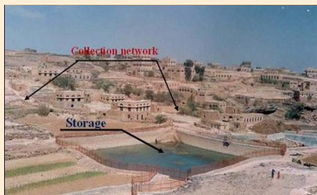
Picture (1.10) Village community water harvesting system
