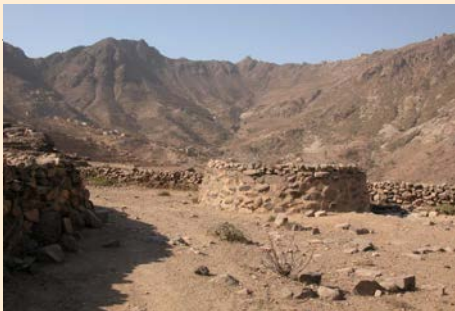
Picture (8.7) Traditional family cistern covered by Qadad roof [19]
