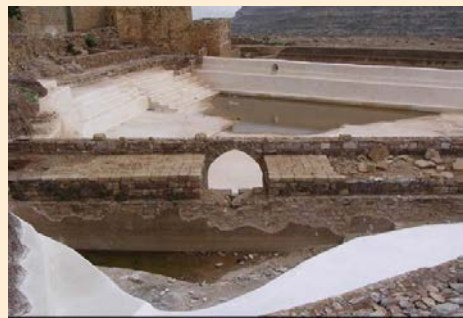
Picture (8.4b) Typical cistern with Qadad plastering in Kokaban city - Yemen
