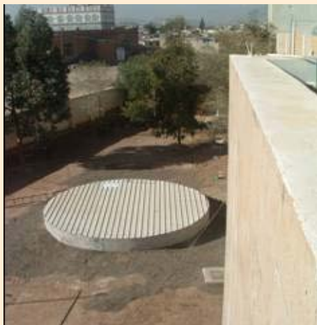
Picture (1.11b) Ferro-cement tank at a girls' school, Sana'a (after completion) (SFD)
