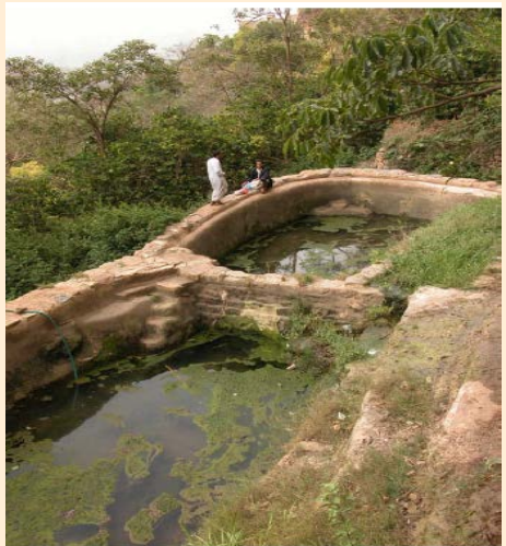
Picture (8.2): Spring cisterns near the city of Hajja [19]
